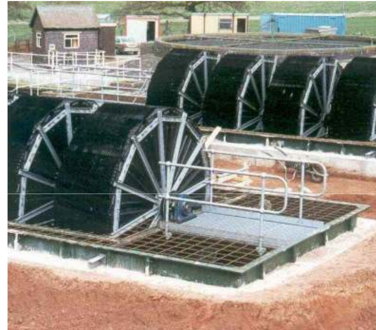
Rotating biological contactor (40% submerged rotates at 1-1.5 rpm)
